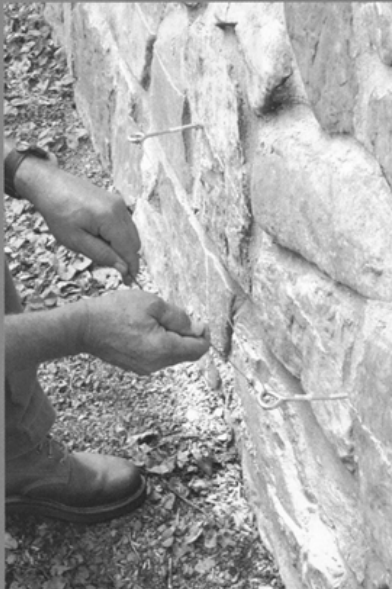
Thread wire through the eye bolts to form a tight network of guide wires.
