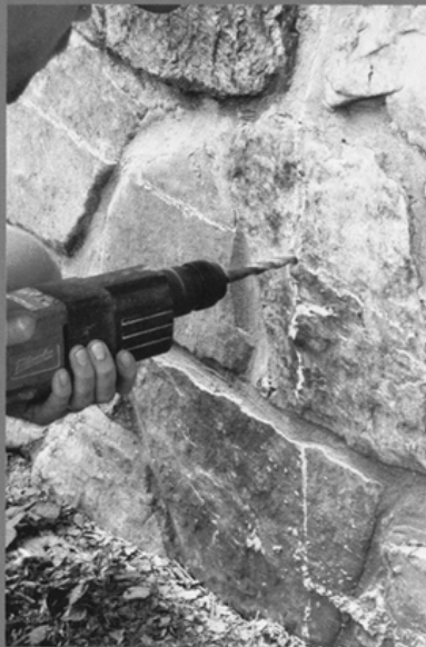
Drill holes 2 inches deep with a masonry bit and insert the lag shields.
