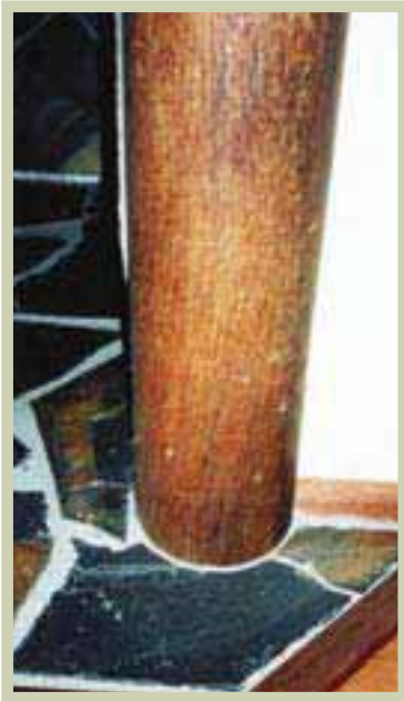
Figure 8-3. An ornamental house post prepared from a coconut trunk. The coconut log was infused with a special wax to impart stability before being machined into this cylindrical post.
