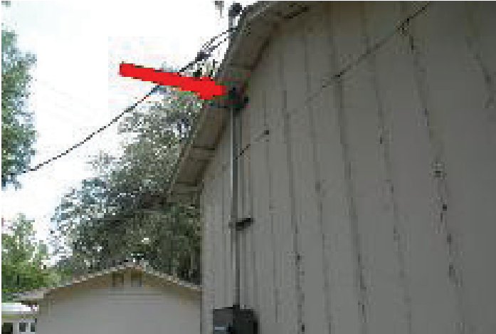
Figure 13. Opening around pipe. Credits: undefined
