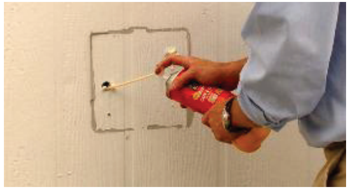
Figure 21. Foaming holes inside of a building. Credits: undefined
