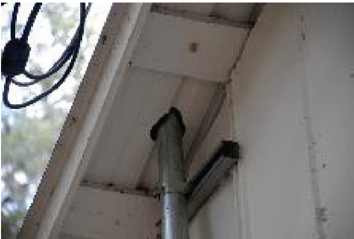
Figure 14. Opening around pipe. Credits: undefined
