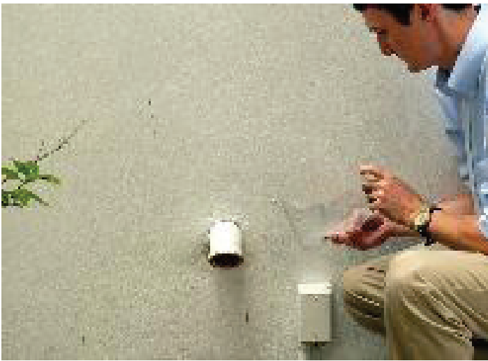
Figure 19. Placing screening over pipe. Credits: undefined
