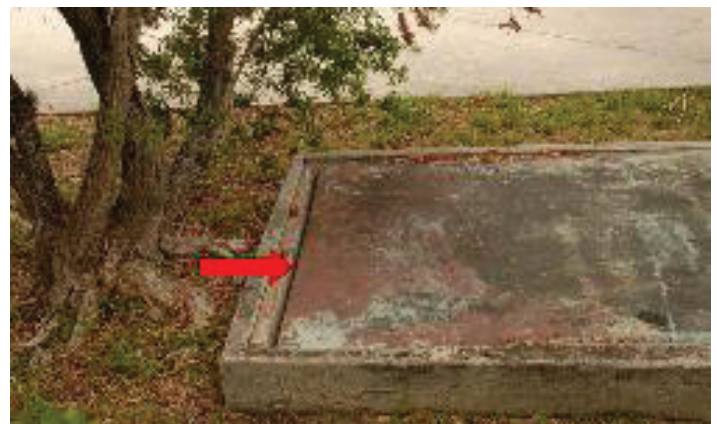
Figure 5. Open space in metal drain cover. Credits: undefined
