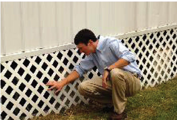
Figure 8. Inspecting under house. Credits: undefined
