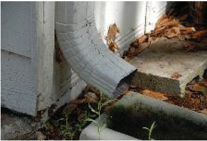
Figure 18. Gutter downspout. Credits: undefined
