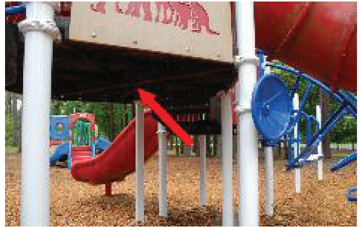
Figure 15. Under playground equipment. Credits: undefined
