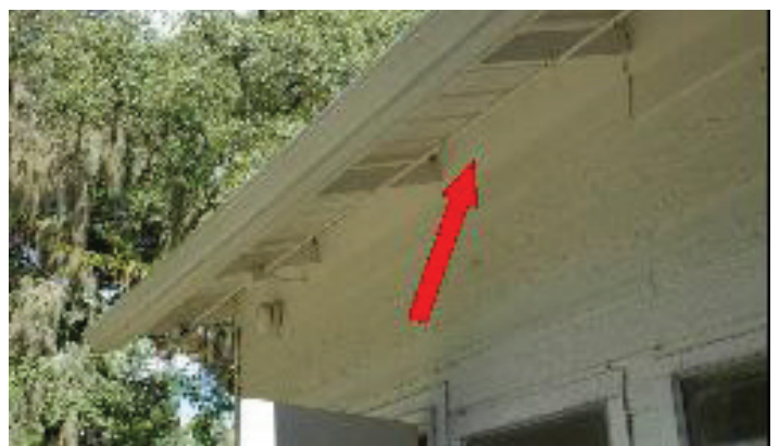
Figure 11. Under eave of house. Credits: undefined
