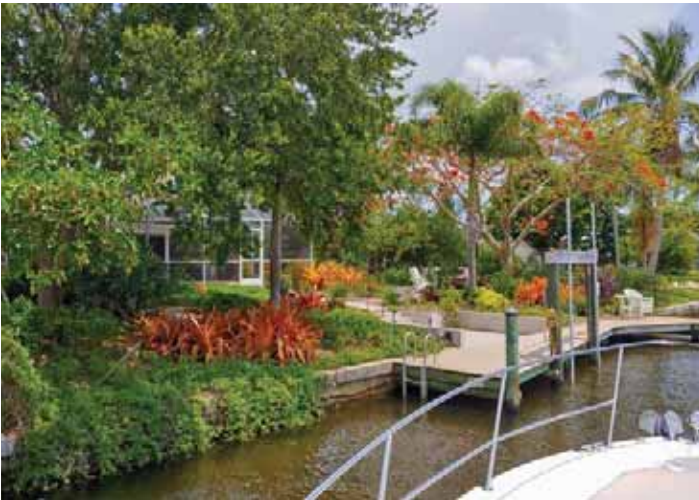
Seawalls can help minimize shoreline erosion but may cause other problems.
