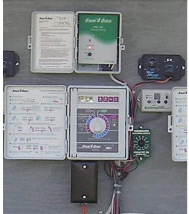
Figure 2. Four brands of soil moisture sensor controllers with an electronic time clock.
