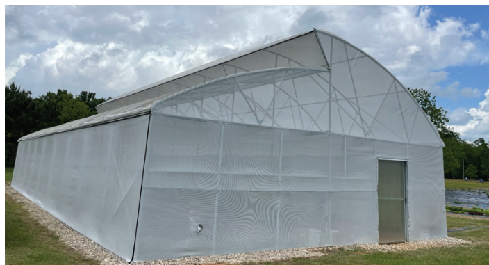
Figure 6. A high tunnel-like tropical screen house structure with a top-vented and poly-covered roof used for protecting crops from excessive rain in Quincy, FL. Credits: Shufang Tian, UF/IFAS
