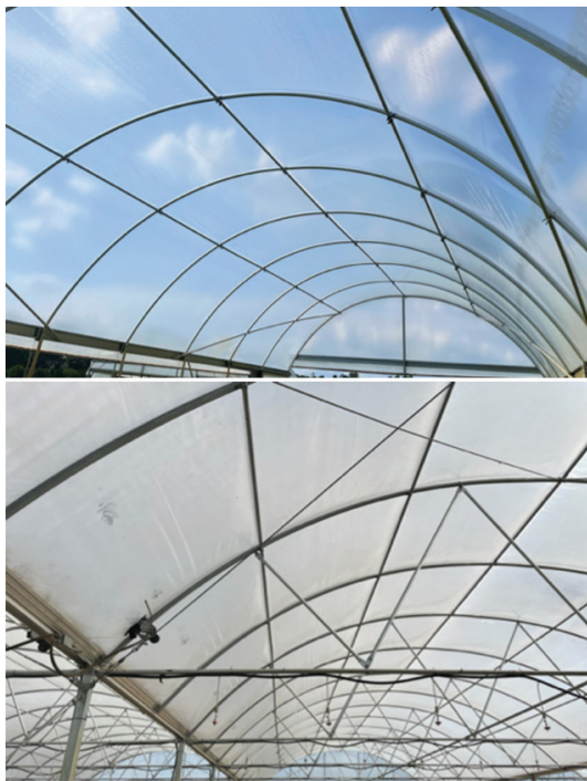
Figure 5. High tunnels covered with a single layer (top) vs. double layers (bottom) of polyethylene film. Credits: Shufang Tian, UF/IFAS
