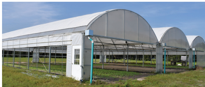
Figure 3. Multi-bay high tunnels.
