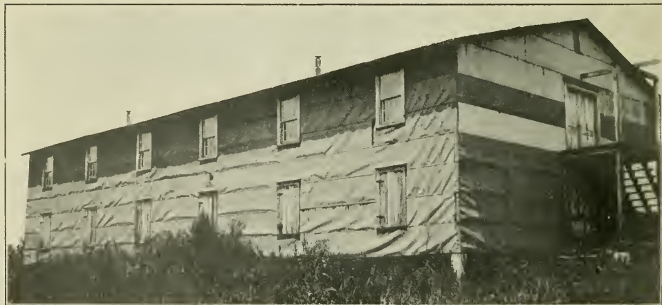
A Community Storage House.
